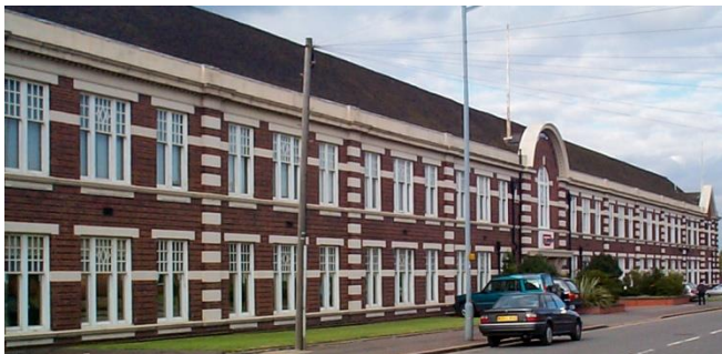
The imposing 400ft frontage of Bromford House, the administrative block fronting the so-called Ward End Works at Drews Lane, in the Washwood Heath area of Birmingham: the home of Wolseley from the late 1920s until the end of 1948.
